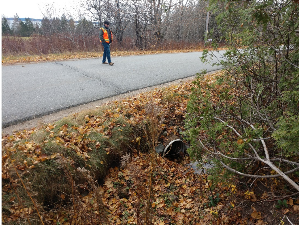
3. 24" CMP culvert crossing Shore Road north of existing driveway
