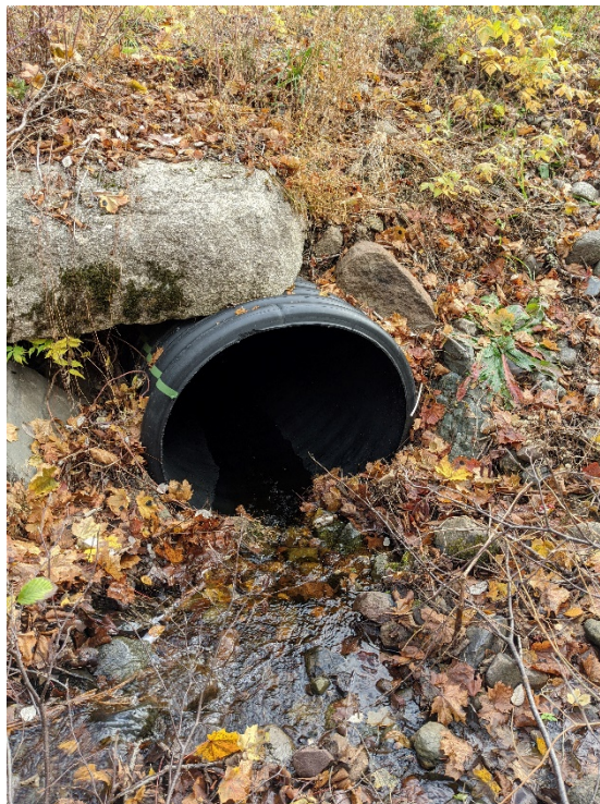
4. 36" HDPE culvert crossing Shore Road south of existing driveway
